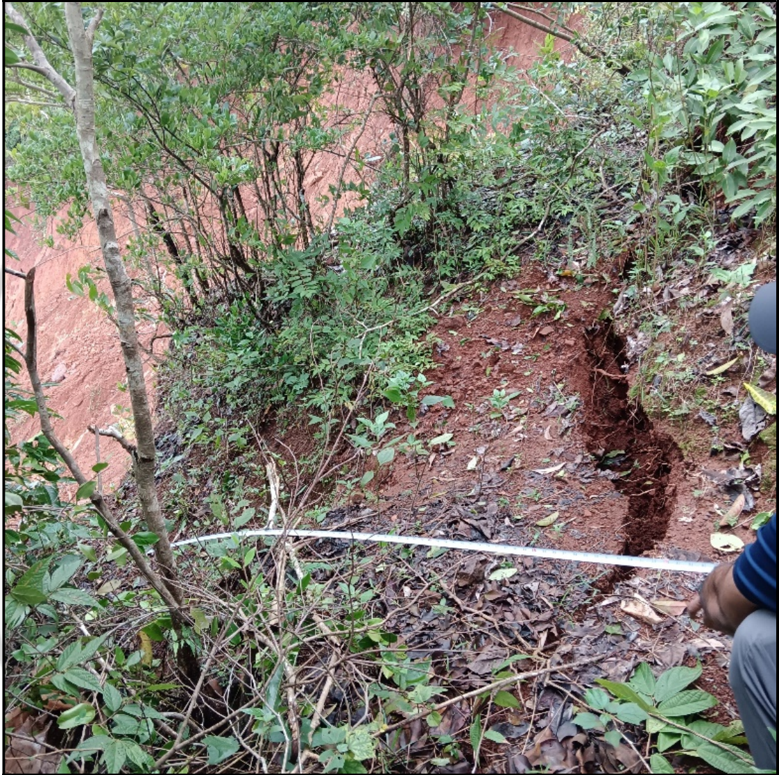
Fig. 1.10: Tension cracks behind the side scar of the slide trending N120°
