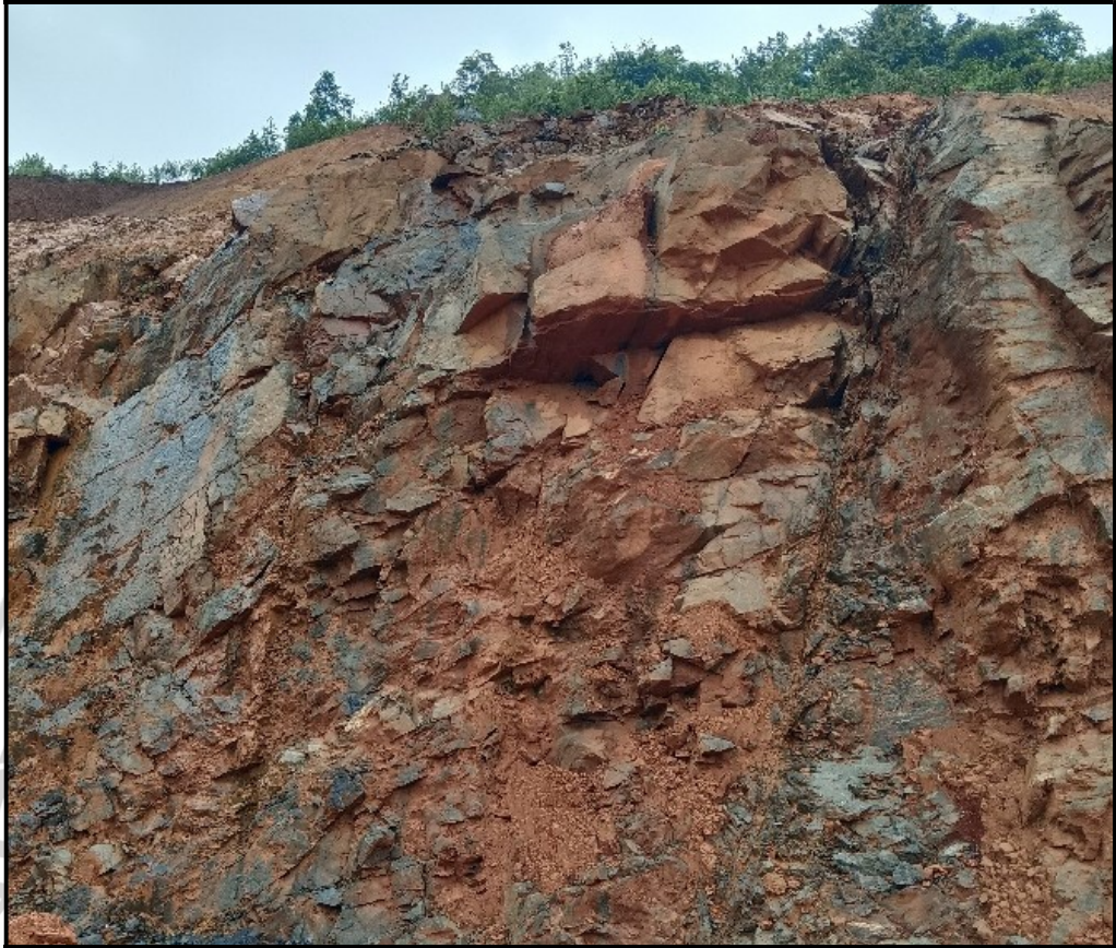
Fig. 1.3: Pyroxenite exposed at the base of cut slope section near Shirur landslide
