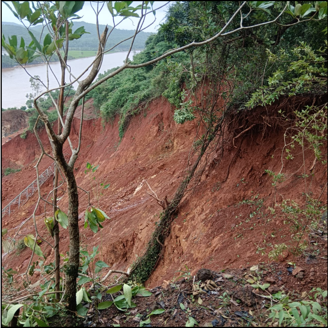
Fig. 1.13: Thickness of overburden at the main scarp
