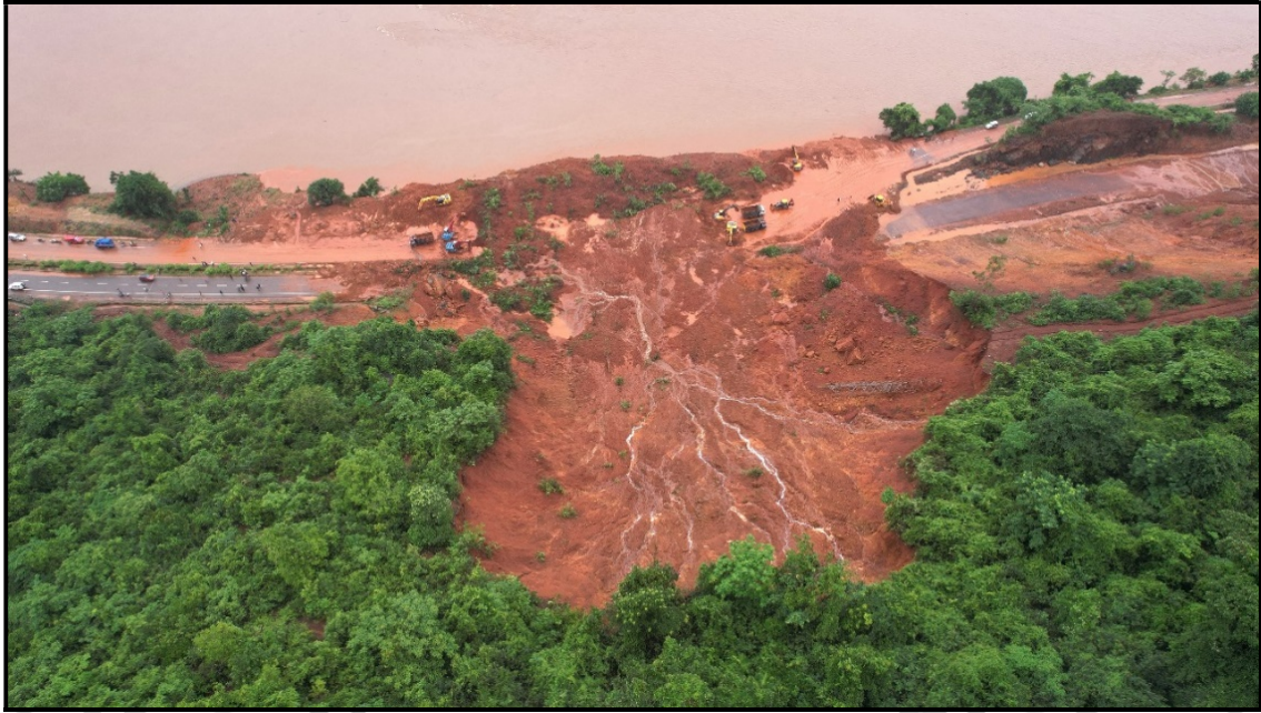
Fig. 1.2: Aerial view of Shirur landslide blocking the communication corridor NH-66 (courtesy IRB)
