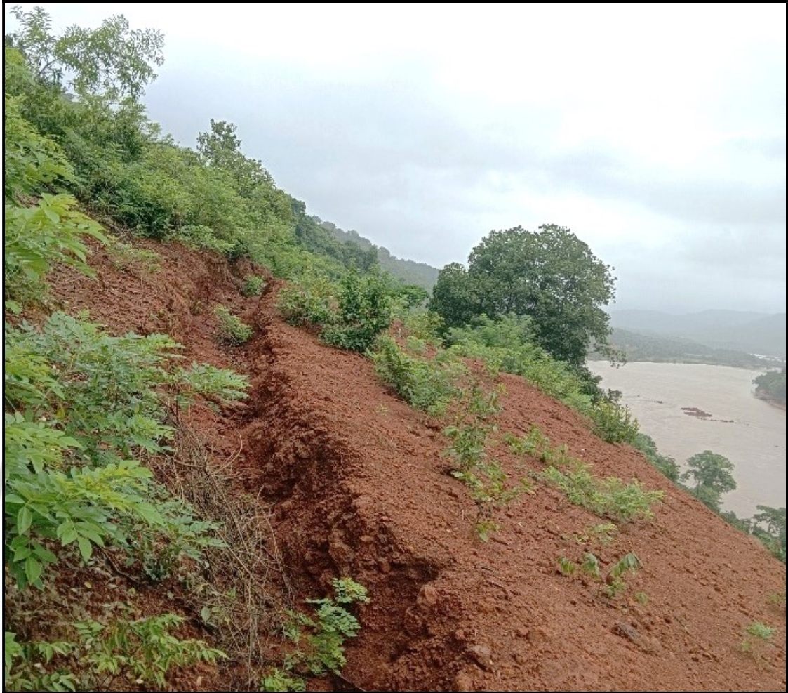
Fig. 1.15: Trenches observed above the Ch. no. 147.500
