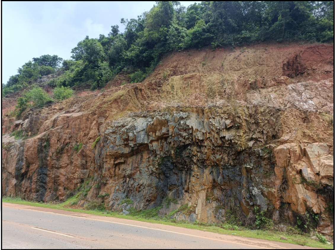
Fig. 2.1: Typical cut section in the sector showing rock-debris interface
